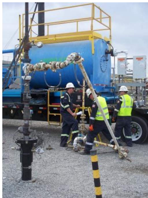
Praxair technicians make adjustments to the CO 2 piping. The injection well itself is in the foreground, left. Photo courtesy Boise Inc.
