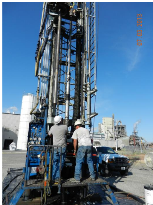
Technicians align a downhole packer and pressure/temperature monitoring system into the CO 2 injection well. Photo courtesy Energy Solutions Inc.
