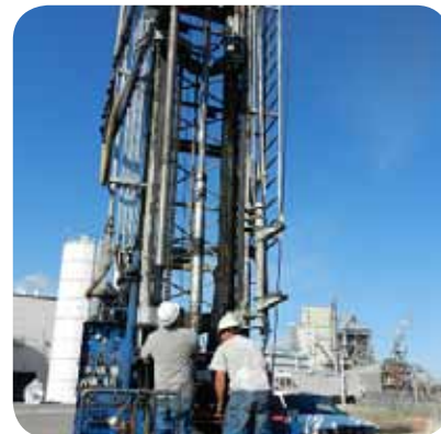
Basalt project injection site, Wallula, WA
